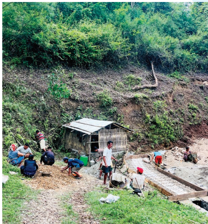
Community members actively involved in the construction of gutter and collection chamber
